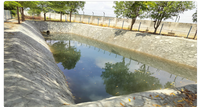
Top: Sewage Treatment Plant installed at Ather factory.
